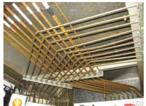
Tungum tube lines after 26 years on Rockwater 1
