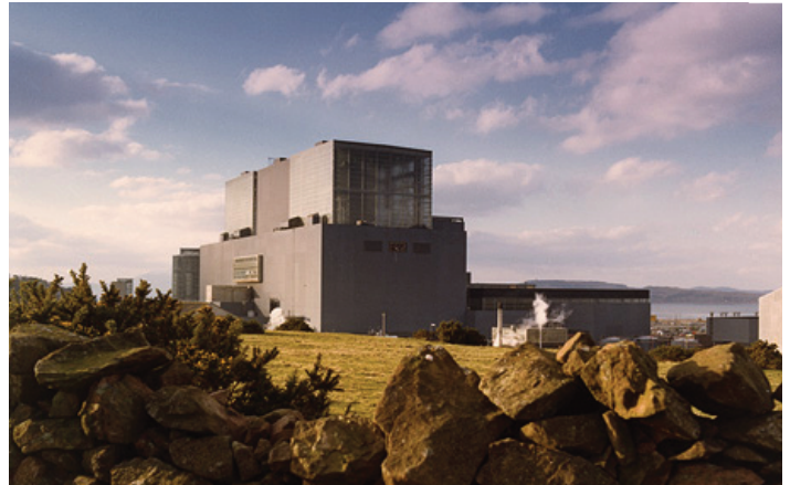
Tungum tubing installed in the Hunterson B
